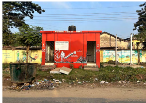
A public toilet complex with poor maintenance in Udaipur, Tripura
